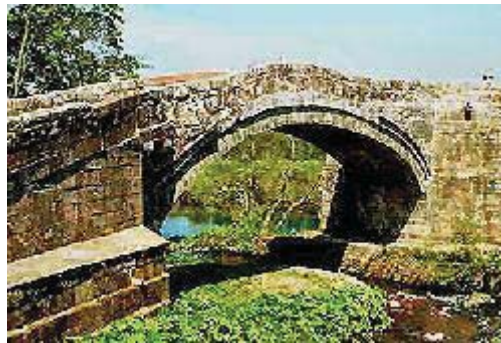
Bridge with elliptical
